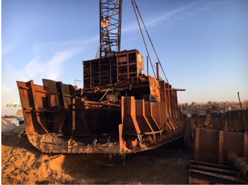
6 February image of the starboard side of Auxiliary Machinery Room being lifted free of the beach.
