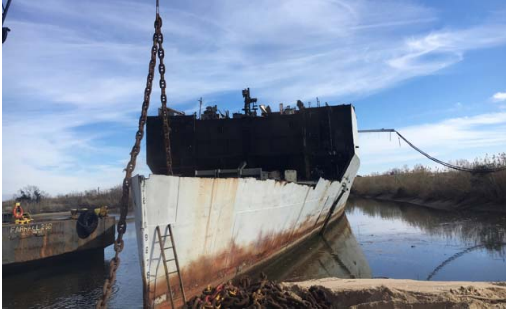
EX-SHADWELL's anchor chains are removed from the chain locker after 1 st and 2 nd Decks have been removed from the bow.
